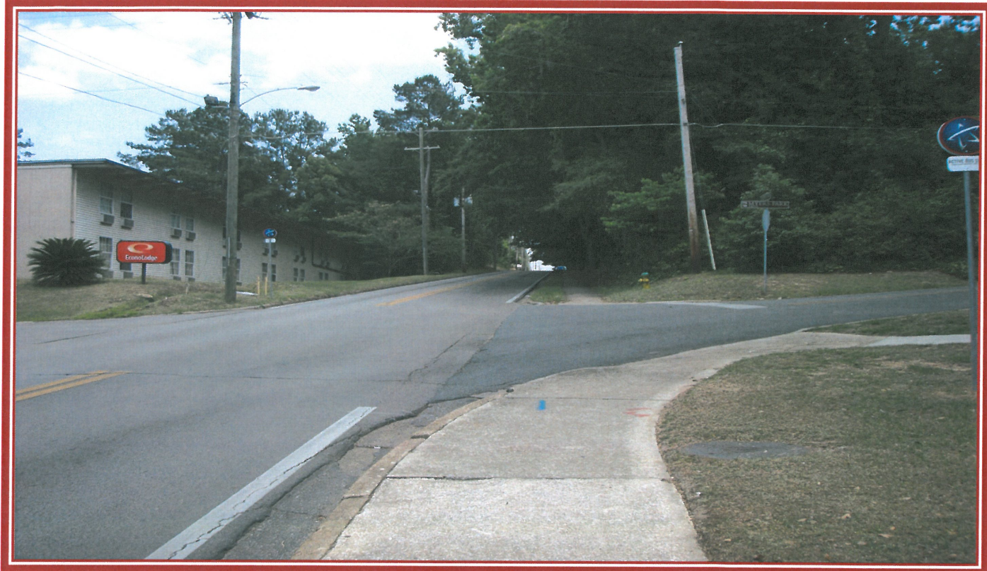
FIGURE 3: PHOTOGRAPH OF EXISTING SITE CONDITIONS (LOOKING EAST)
